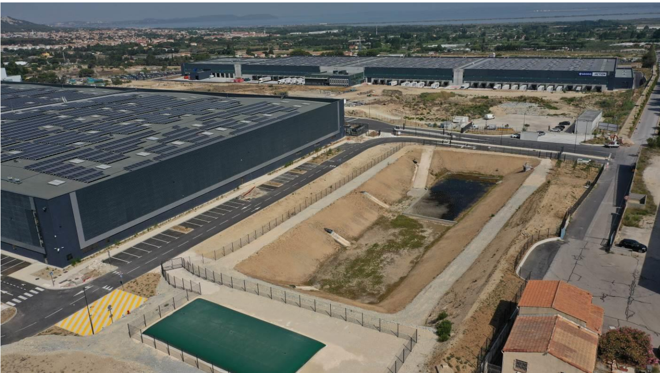
Figure 80 : Bassin – lot H
