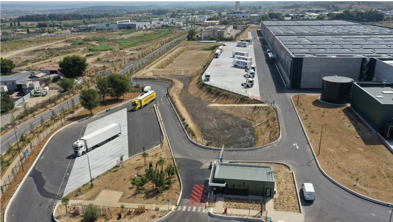
Figure 79 : Bassin – lot D
